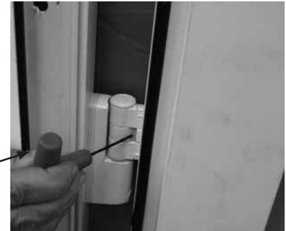
This will release the hinge cover.
