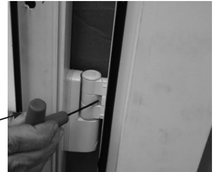
This will release the hinge cover.
